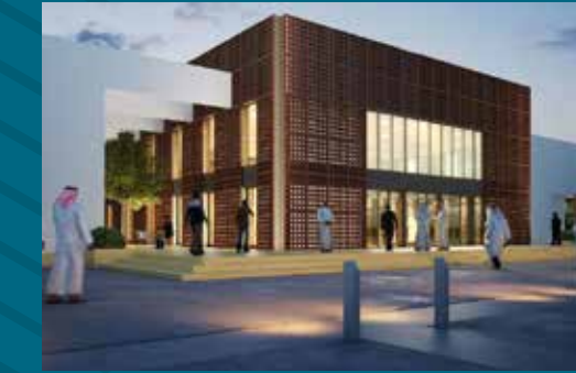
QATAR UNIVERSITY ANNEX BUILDING MEDICINE COLLEGE
